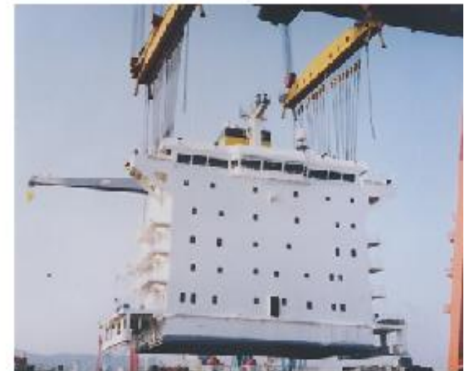
Fixing superstructure
